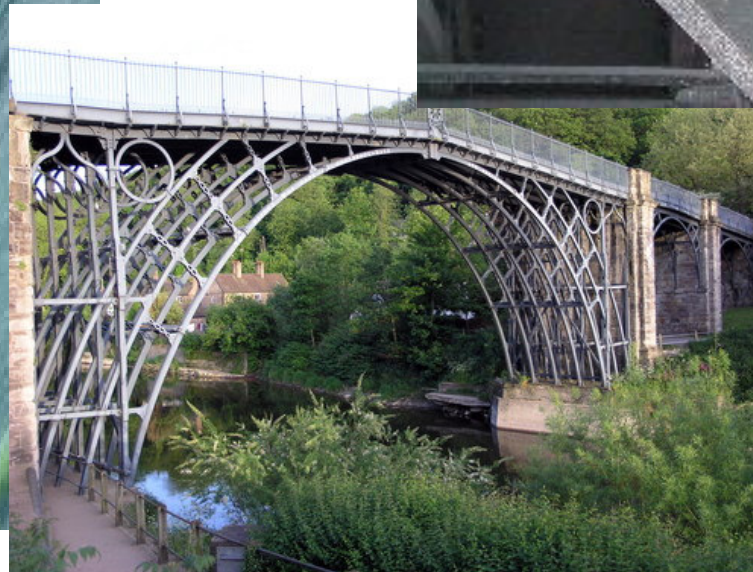
The world's first bridge made of iron in 1779. The entire structure is made of cast iron. (near Broseley, UK)
